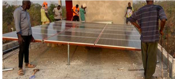
INSTALLATION OF SOLAR PANELS
